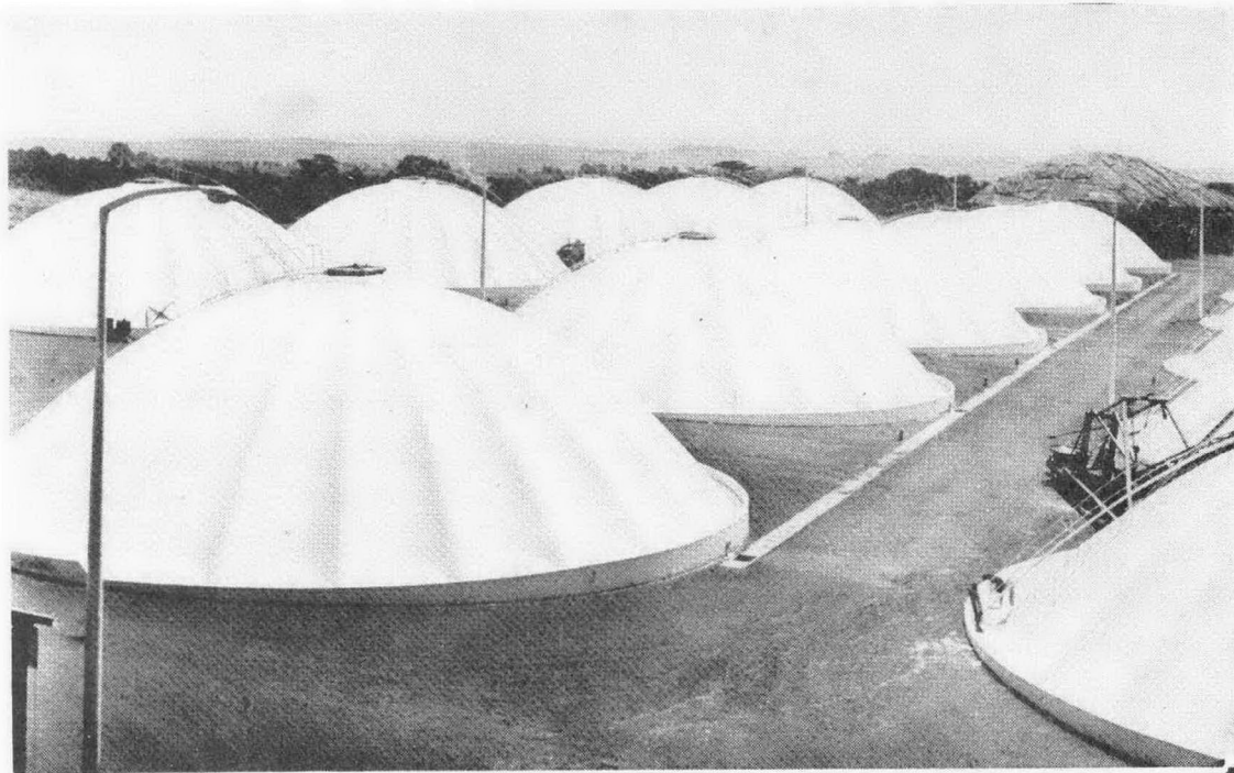
Figure 2. The "Cyprus Bins" - semi-underground hermetic structures. Each bin can hold approximately 1,500 tonnes of grain.
