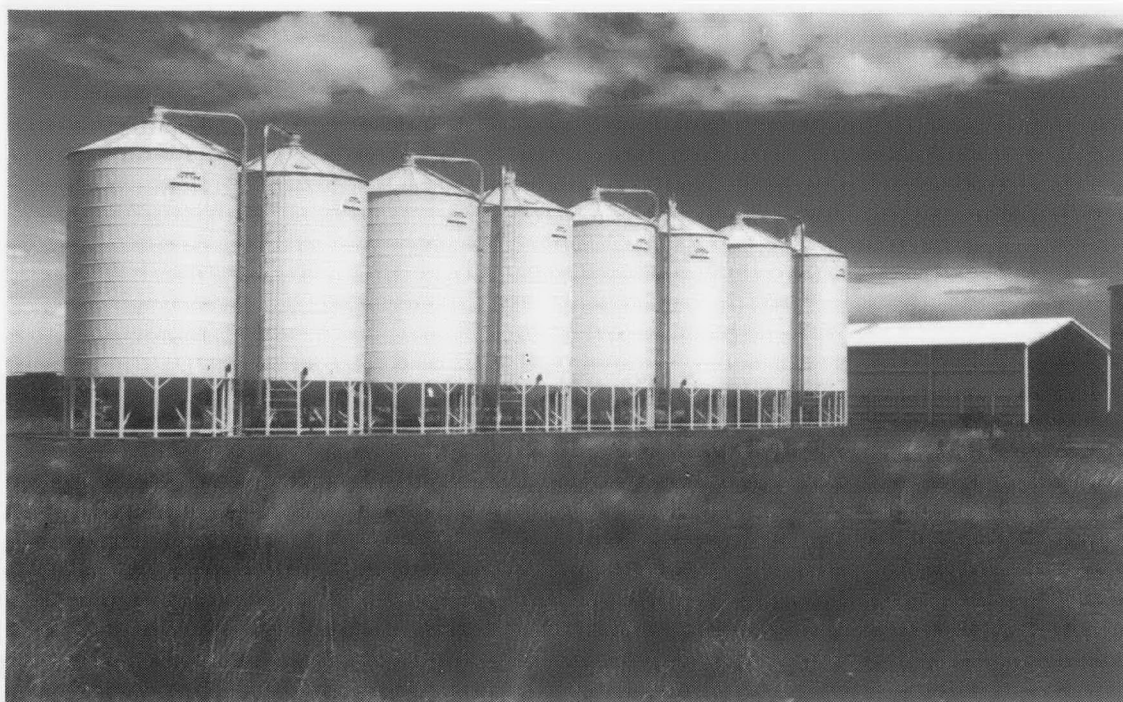
Fig. 11. An on-farm bank of 140 m 3 hybrid silos incorporating several grain management and handling features: — sealable for fumigation or CA; white Colorbond® construction for temperature stability; pneumatic filling; provision for aeration equipment.
