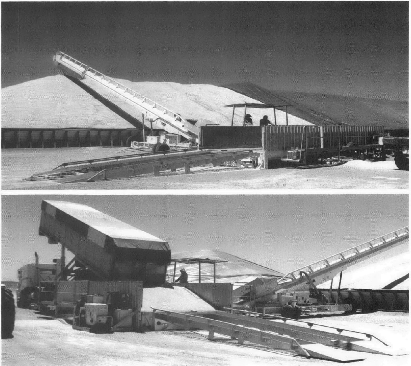
Fig. 1. Mobile drive over hoppers and stackers for filling and emptying grain bunker storage
