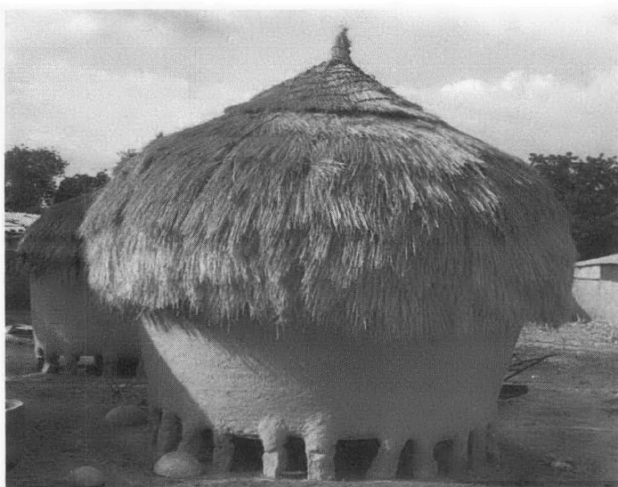
Fig. 6. (a) Above: rhumbu with thatched roof elevated on stones to guard against rodents. (b) Top right: rhumbu with opening for easy access to grain. (c) Lower right: rhumbu built as part of house wall (protection against intruders).
